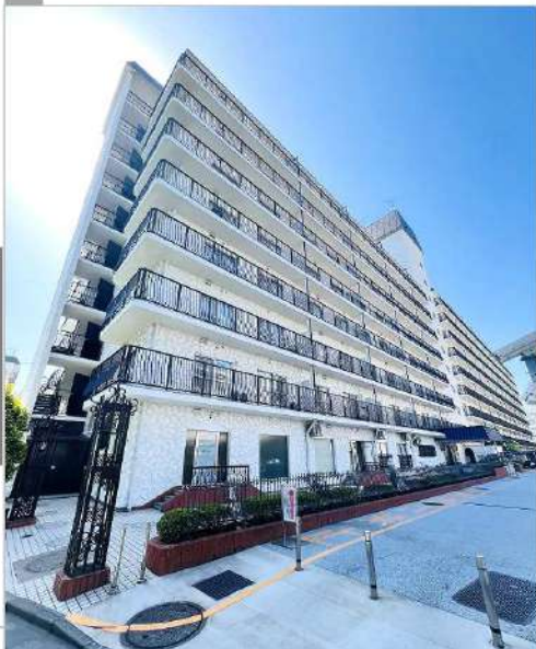
SYUWA Hatagaya - Residence
